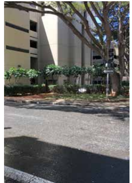
Crosswalk next to City-owned residential towers is invisible
