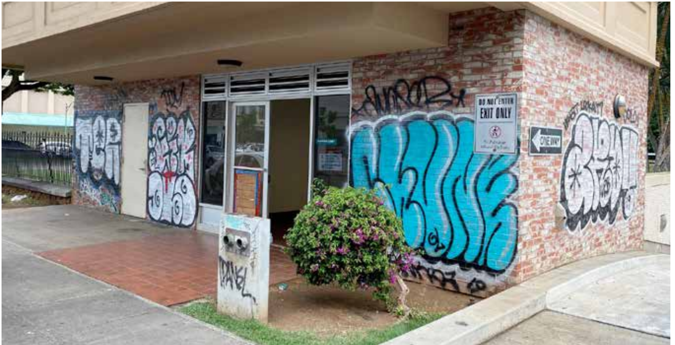
City-owned elevator building at Smith Beretania Park
